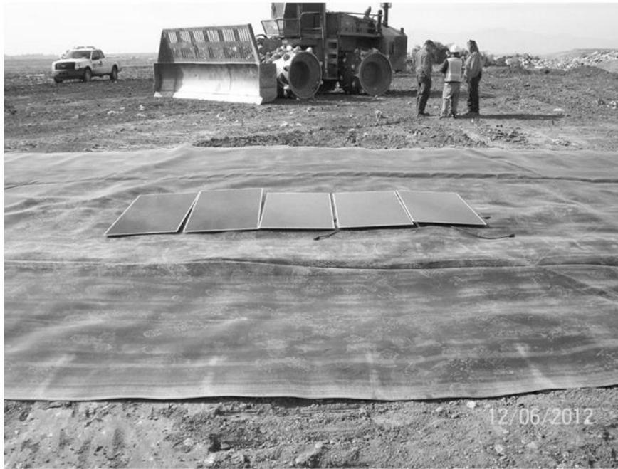
Figure 2. Aljon model 91K compactor used to crush CdTe PV modules in a Municipal Solid Waste Landfill in the State of Arizona, USA.
